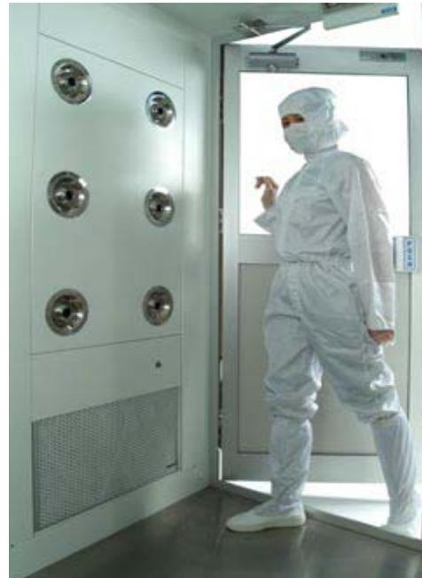
To enhance cleanroom integrity, there is a pre-purge period set to activate the fans when the air shower is just turned on. Users can choose to bypass the pre-purge by setting the duration to 0. The default duration is 10s while the maximum duration is 3 min.
